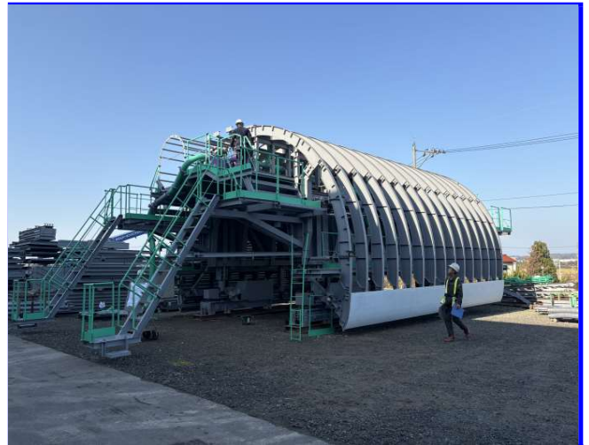
FRP型枠組立①
